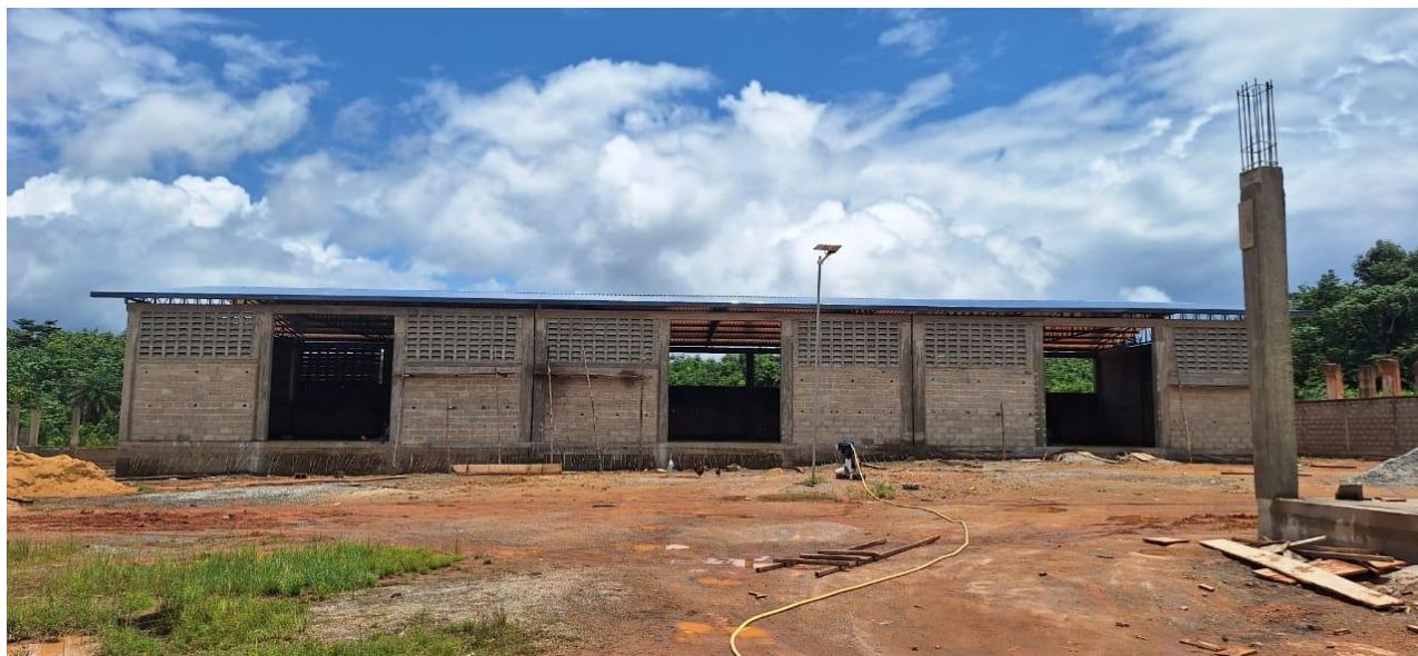
The Dupkuyee Wood Workshop currently being constructed in Dupkuyee Township, Nimba County, Liberia
