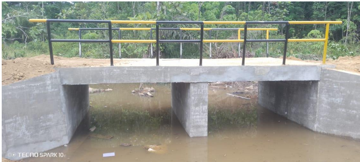
One of the two box culverts constructed by GoL and implemented by LACE in Kpo Township, Todee District, Montserrado County, Liberia
